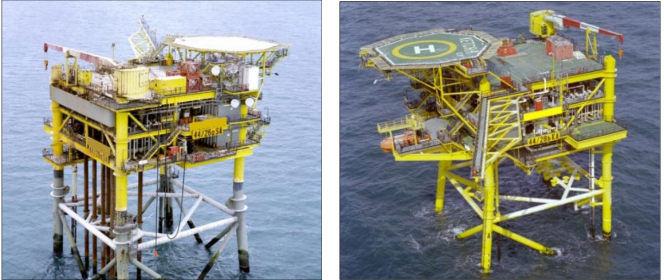
Figure 2: Schooner and Ketch Normally Unmanned Installations (NUIs, Ketch was removed in 2022)
